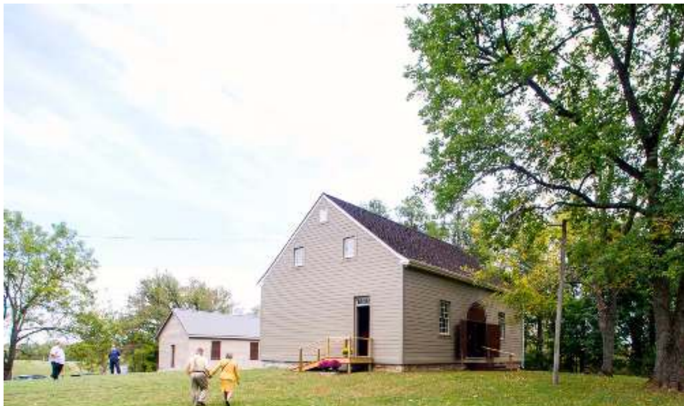
Figure 16: The restored Old Mud Meetinghouse, and one-room school in 2015. Work continues.
